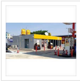
Portable Petrol Pump Offices
